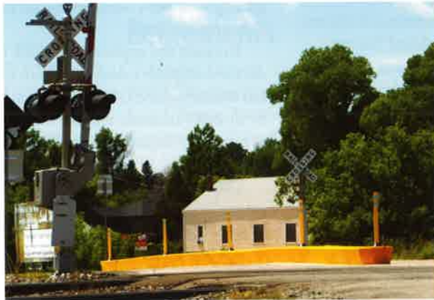
A quiet zone crossing in Lusk utilizing a barrier median in front of the gates.
